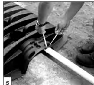
Secure pressure pipe.
