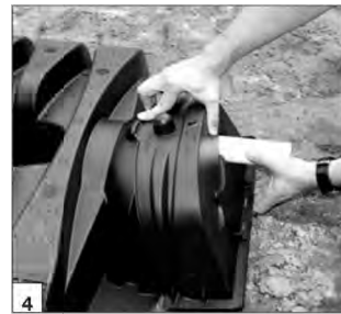
Place end cap over inlet end.
