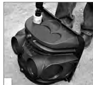
Drill pressure pipe hole.
