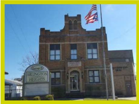
ARLINGTON HEIGHTS MUNICIPAL BUILDING 601 ELLIOTT AVENUE
