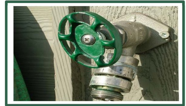
PREVENTS BACK-SIPHONING OF CONTAMINATED WATER INTO HOME PIPING
